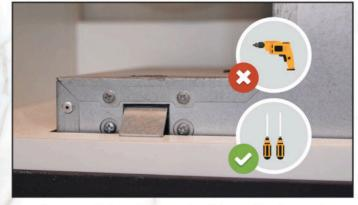
**STEP 6:** To avoid the clip from breaking easily, please do not tighten it with **electric drill;** use only **screw driver** to tighten it.
